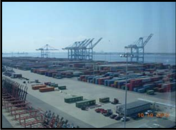
Cranes in the background and cargo containers offloaded and stored by GPS location
